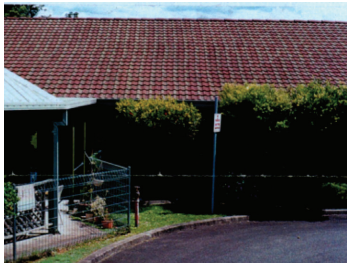
Photograph 6 – Distorted rows of roof tiles and trusses due to inadequate roof bracing
