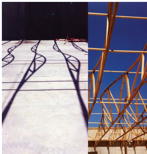
Photograph 10 – A pronounced example of incorrect installation leading to trusses being twisted and out of plumb
