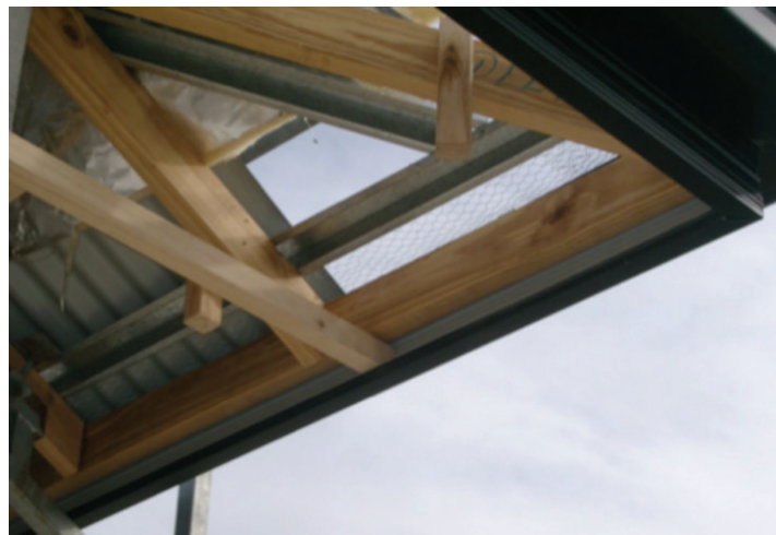
Photograph 9 – Ensure structural fascias are installed in accordance with the truss design and specifications
