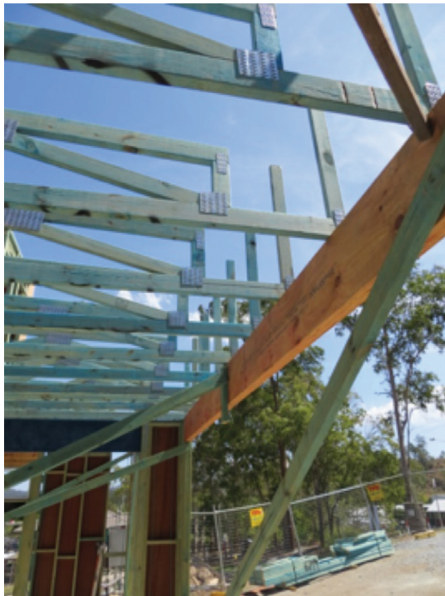
Photograph 11 – Structurally deficient parapets
