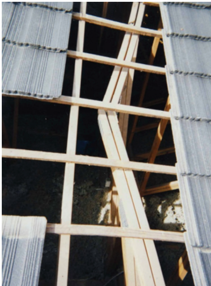
Photograph 5 – Inadequately fixed roof battens resulting in lateral buckling failure of girder truss
