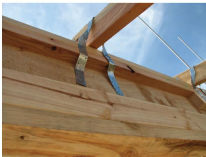
Photograph 10 – Truss tied direct to top plate and lintel, but strap bent through too great an angle to be effective
