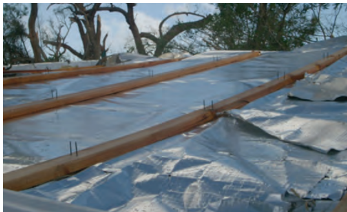
Photograph 5 – Roof sheeting and battens have failed due to nailed batten fixing where screws should have been used
