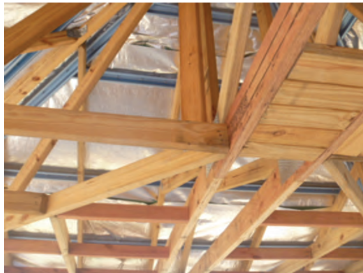
Photograph 8 – Inadequate connection of jack and hip trusses to girder truss for a C2 wind classification
