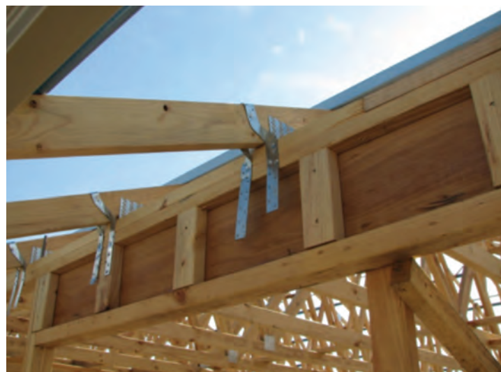
Photograph 9 – Incorrect practice for tying down over openings as top plates not tied to lintel
