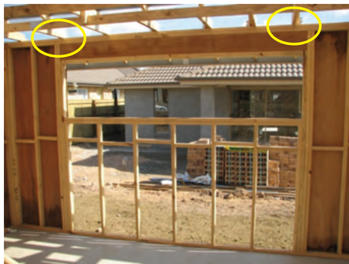
Photograph 11 – Plywood cannot be used to effect tie-down at sides of openings as the trusses highlighted above must have 300 mm min of ply to the right and left side respectively
