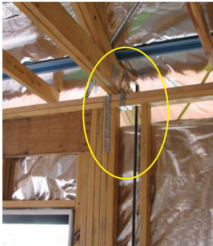
Photograph 7 – Double straps connecting girder truss to top plate and jamb studs (strap to jamb stud should have been centrally located on stud). Cyclone rod correctly located within 100 mm of truss tie-down
