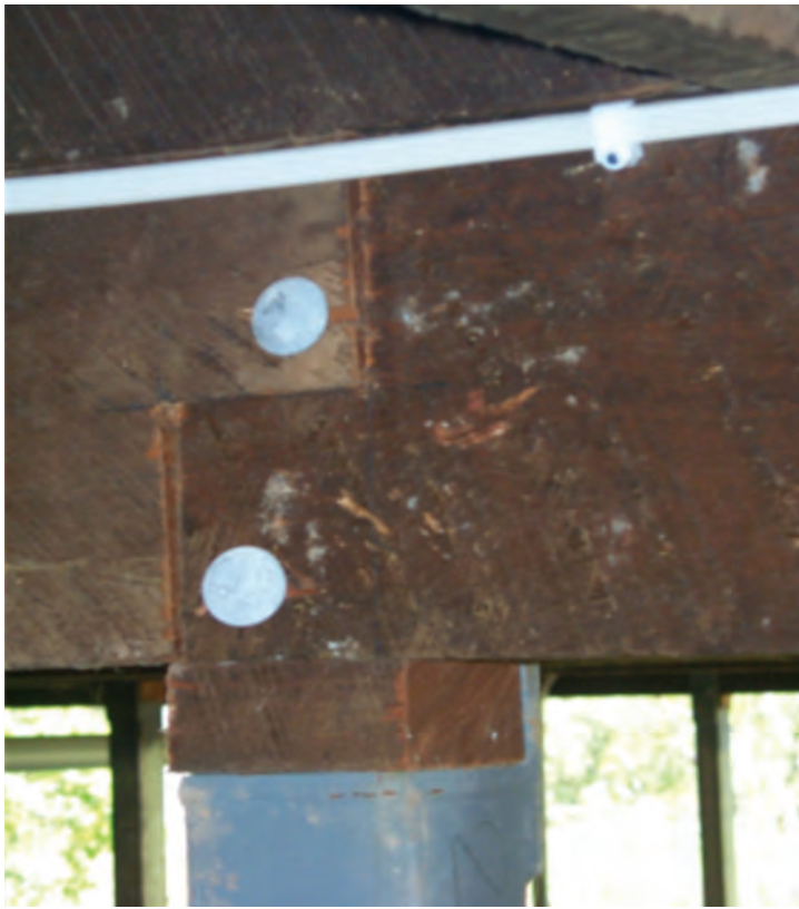
Photograph 15 – Minimum bolt end distances less than required to achieve uplift capacity. Also, unseasoned timber packer used is not suitable due to shrinkage
