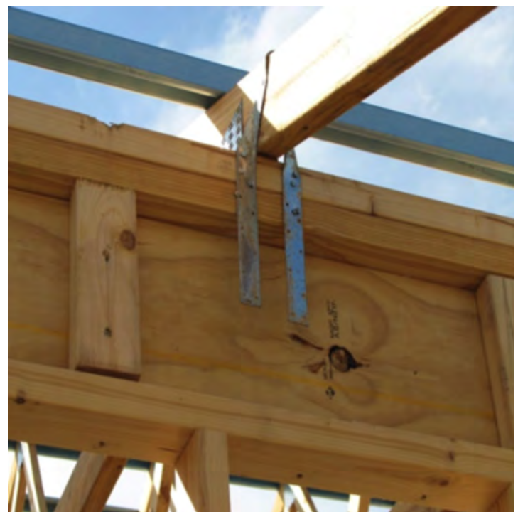
Photograph 1 - Inappropriate practices as nails are too close to strap edge, too close to pre-punched holes and even doubled up. Strap should also have been installed on the inside of frame to enable strap nailing direct to lintel without bending the strap
