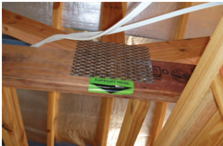
Photograph 6 – Girder truss incorrectly supported by an offset wall
