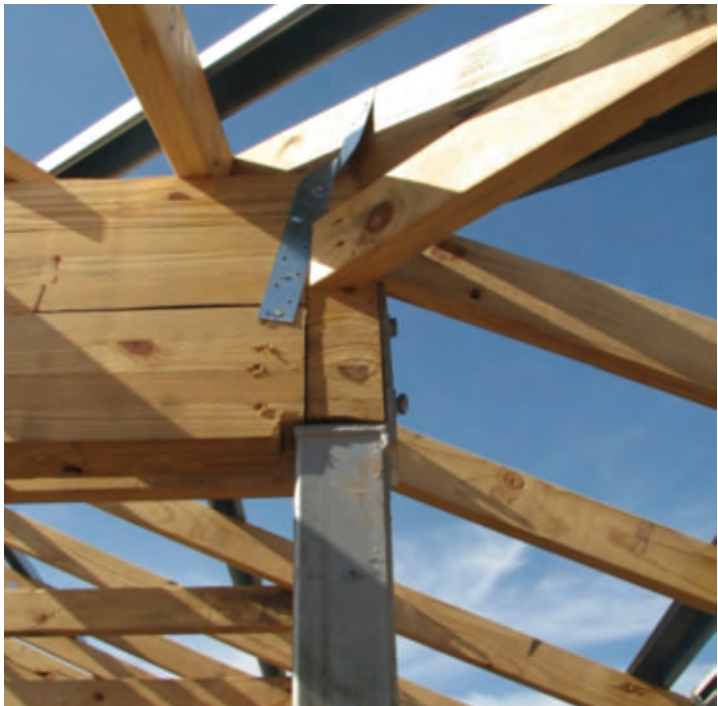
Photograph 16 – Intersecting verandah beams. The LH beam has inadequate bearing and tie-down capacity
