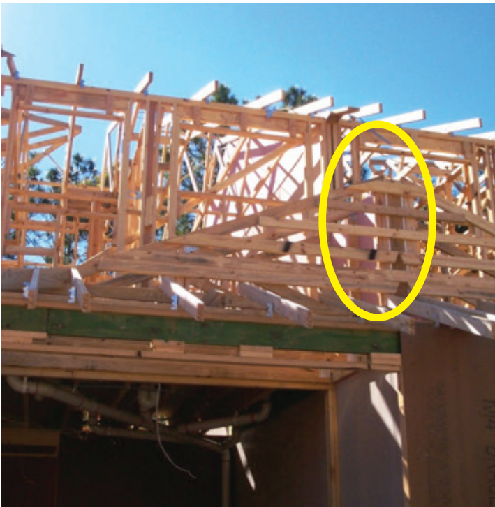
Photograph 3. Separating wall extends out through Dutch Gable, however the framing members that cross the end of the Dutch Gable will not comply with the fire separating wall requirements.
