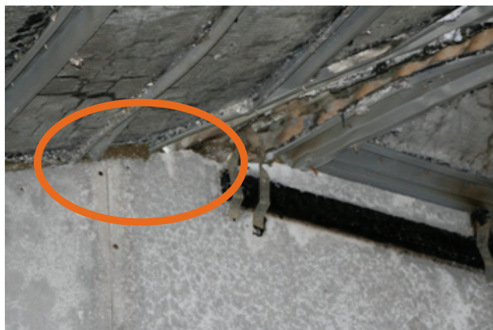
Photograph 1. Fire damaged unit. Note: gaps between battens filled with mineral wool to prevent fire spread across separating wall.
