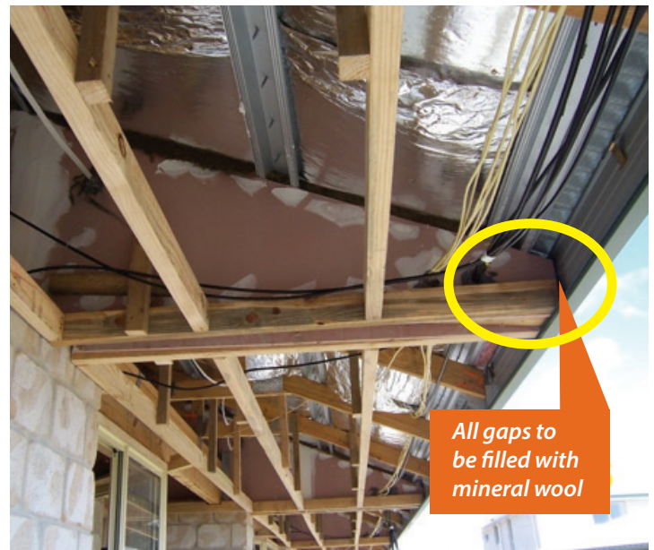
Photograph 5. All spaces are required to be filled with fire resistant mineral wool or other fire rated material including under all top hat battens, behind fascias and to the end of the separating wall.
