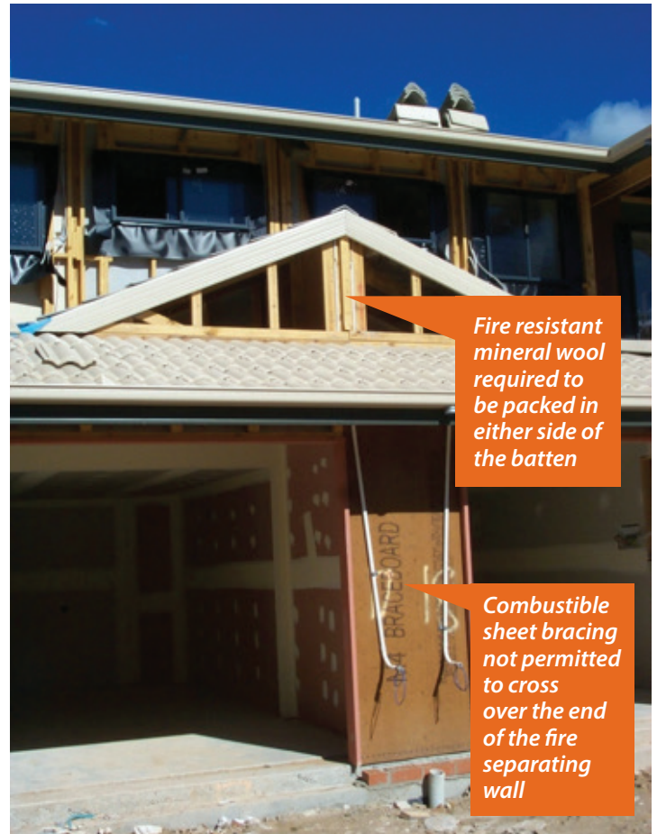
Photograph 4. Separating wall extends out through Dutch Gable. To comply, the vertical batten on the end of the wall will require fire resistant mineral wool to be packed into the end cavity either side of the batten.
