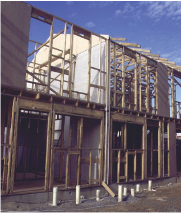
Photograph 2. Fire rated plasterboard extends beyond outside of external wall frame and into cavity. End of separating wall to be fitted with fire resistant mineral wool and DPC.
