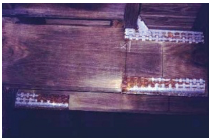
Photograph 2 - NOT ACCEPTABLE – Z275 connectors in deck joists 1 km from surf. 6 years old, Sunshine Coast.
