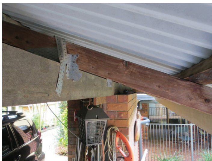
Photograph 1 - ACCEPTABLE – Z275 bracing, multigrips and truss plates in a Low Hazard (>10km from surf) Sheltered Condition. Note: Connectors have been installed for 35 years.
