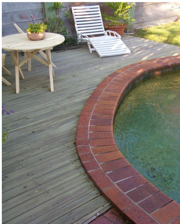
Photo 2: Timber Deck on the Ground - H4 (min) Hazard
