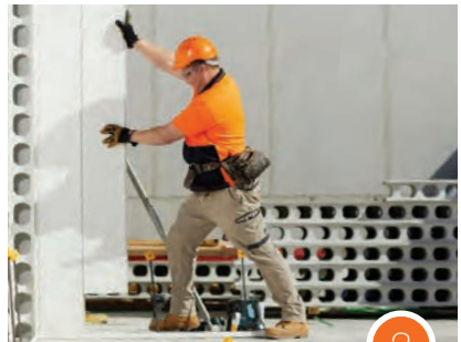
And simply slide down to seat into the floor tracking and form a wall
