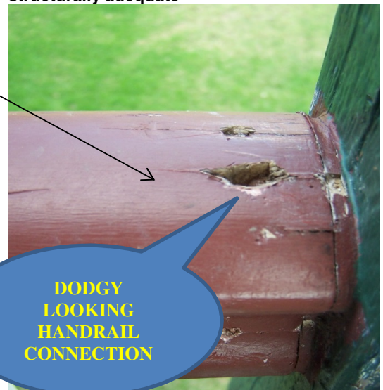
Make sure handrail connections are structurally adequate
