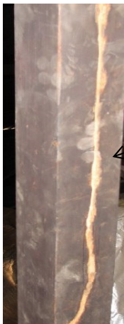
Check the base of posts to ensure termites have not accessed timber above.
