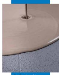
Application of Ultraplan self-levelling smoothing compound on dry Eco Prim Grip on old floor
