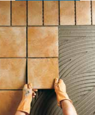
External installation of klinker tiles
