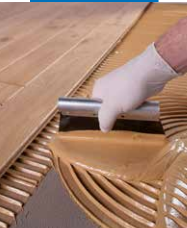
Spreading Ultrabond P990 1K
