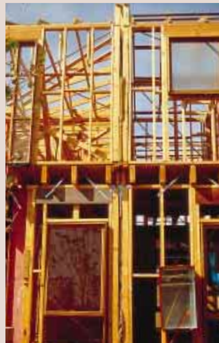
Double stud separating wall system between townhouses.
