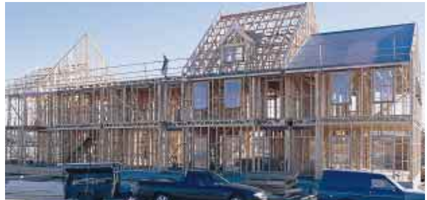
Speed of construction is easily achieved with full timber framed construction.
