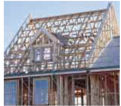
Speed of construction is easily achieved with full timber framed construction.
