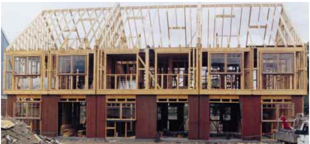
Fire & sound-rated timber framed separating walls (party walls) offer acoustic superiority at a lower cost.
