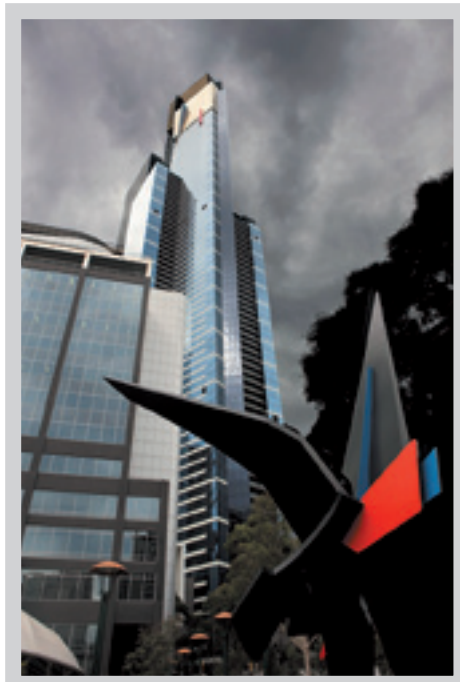
Level 89 Function Centre, Eureka Tower, Melbourne
